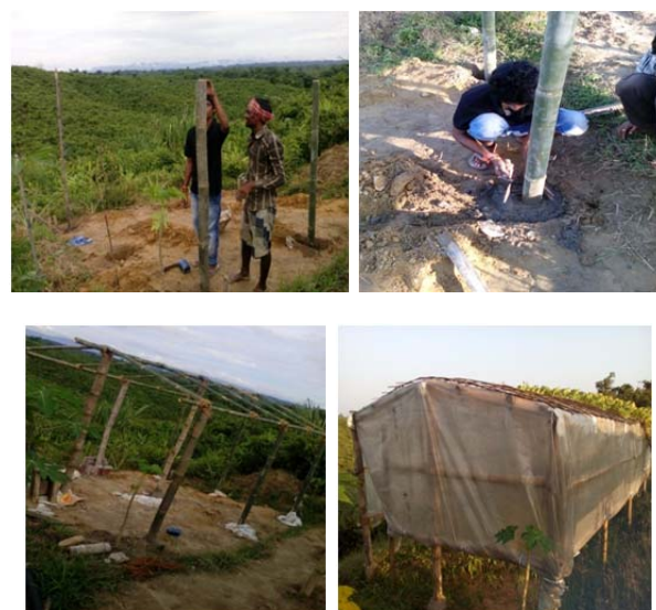
Plate 1 A View for Construction of Low-cost Poly House
